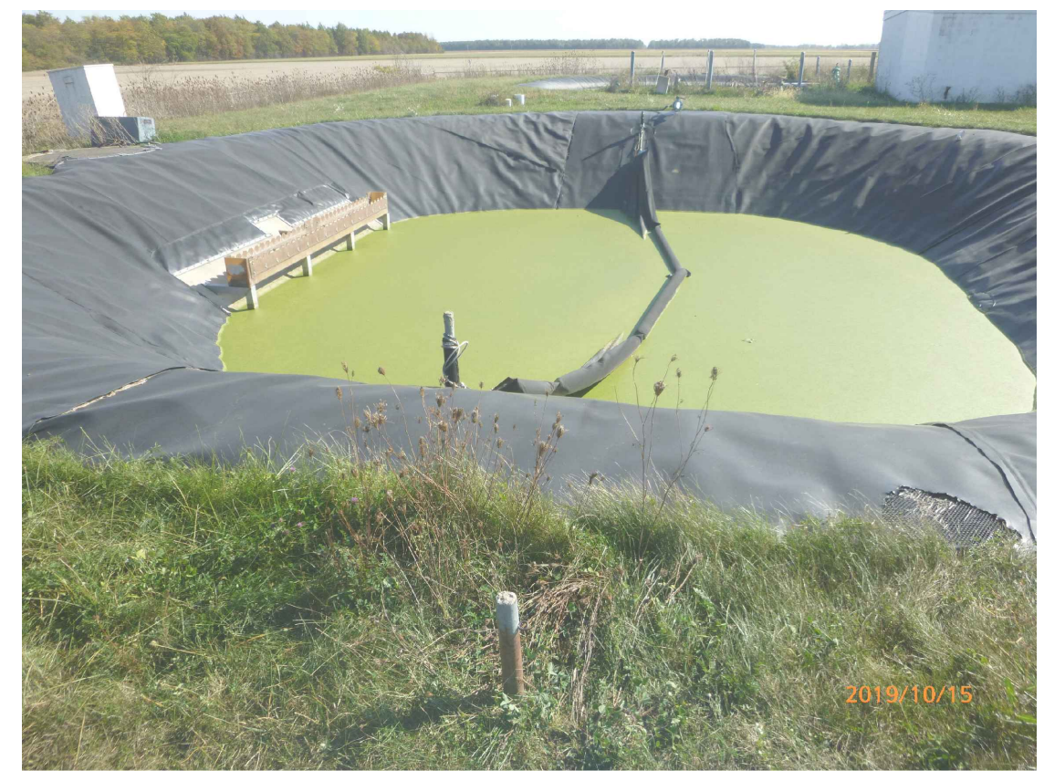
EXISTING POLISHING BASIN: FLOATING FABRIC BAFFLE & EFFLUENT TROUGH
