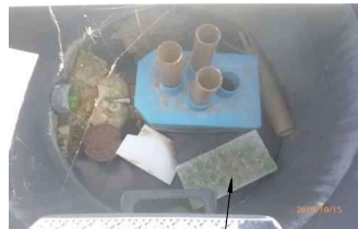
DEMO EXISTING CHLORINATION EQUIPMENT AND CLEAN STRUCTURE. INSTALL BENCH AND CHANNEL.
