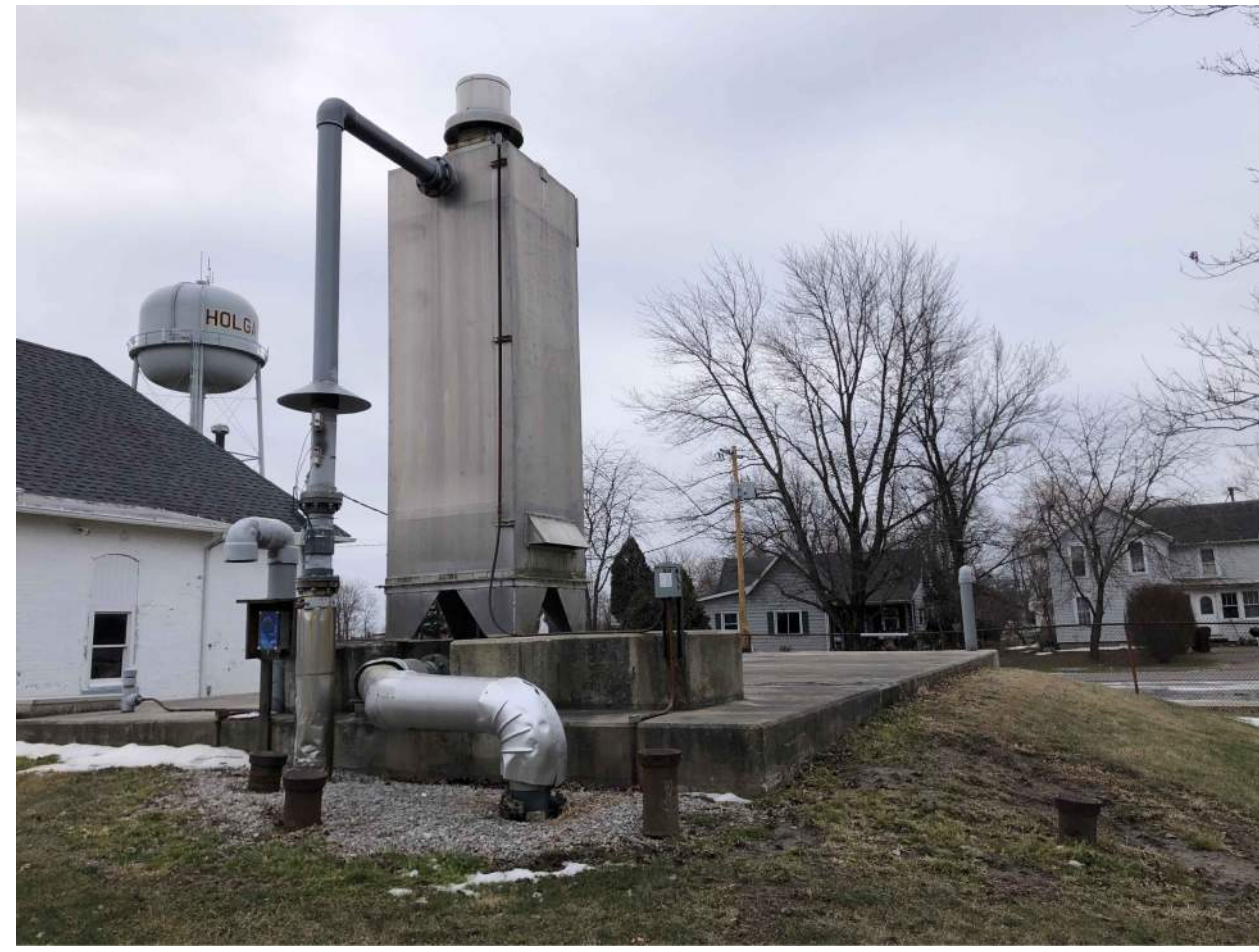
EXISTING WELL NO. 1 AND AERATOR SCALE: NONE
