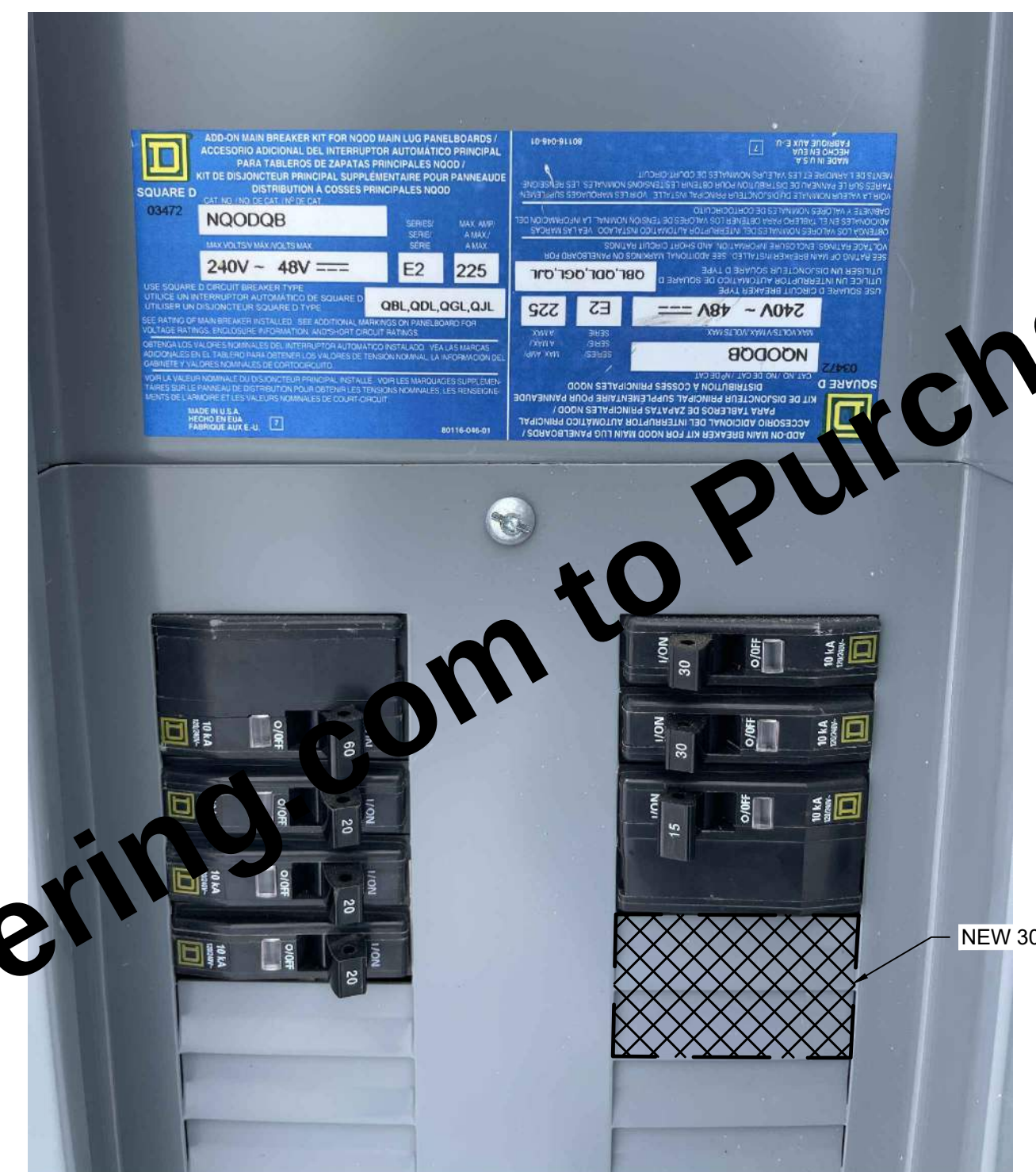
EXISTING 120/240V PANELBOARD MODIFICATION SCALE: NONE
